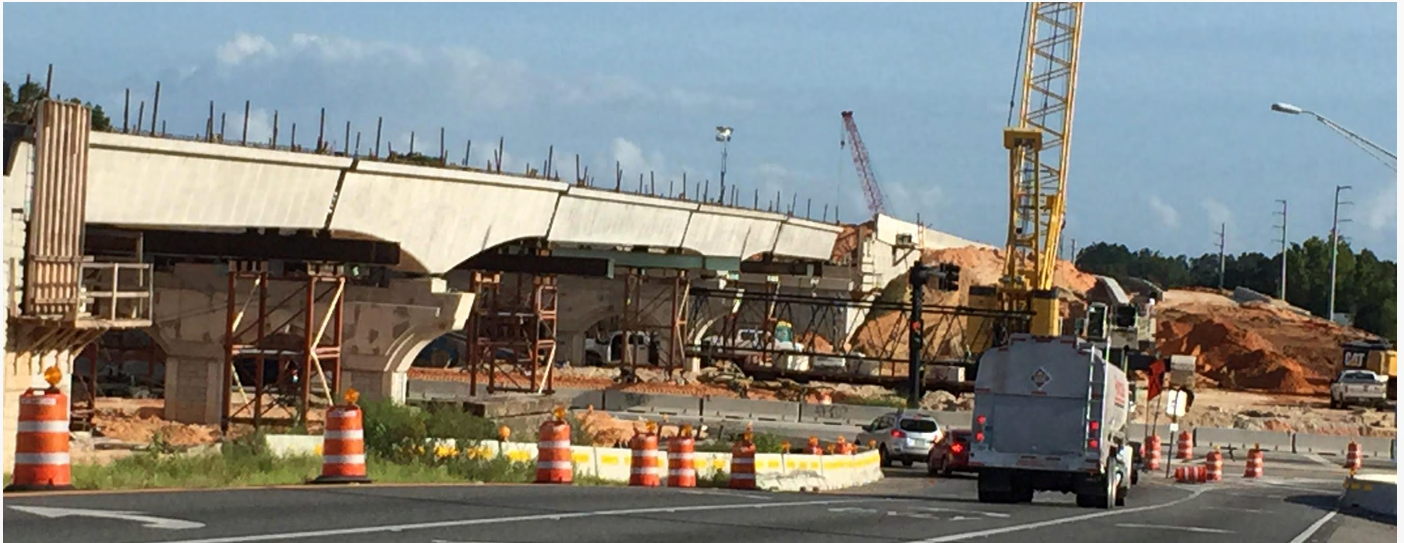
SR 429 Connector Road Bridge - 30, 100 Ft. Beams in Place
