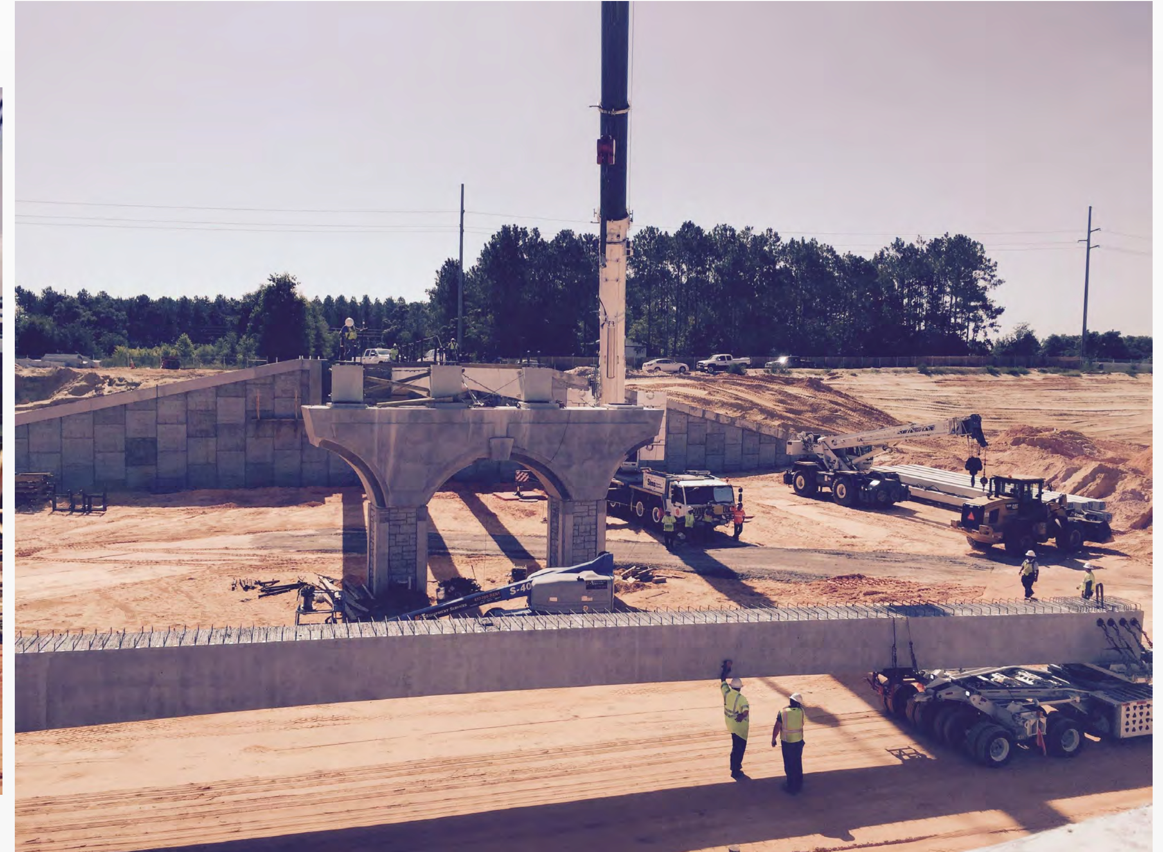
“Depressed” Section at New Belgian Street Bridge
